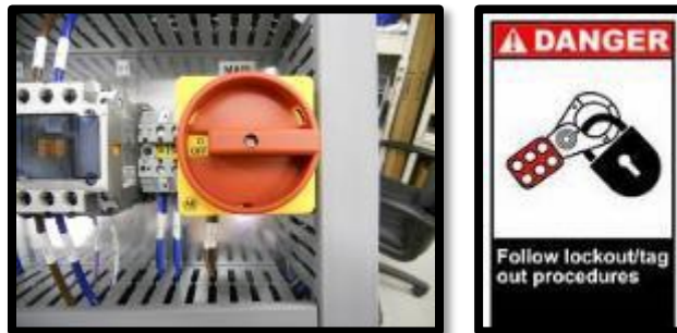
Figure 5, Main Disconnect
