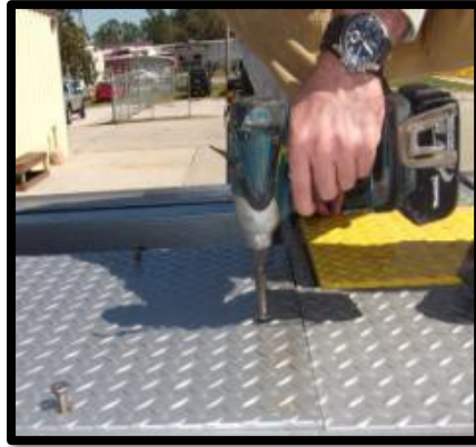
Figure 4, Remove Top Plate Screws
