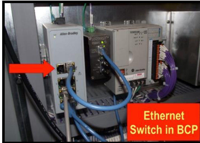
Figure 8, Ethernet Connection at BCP
