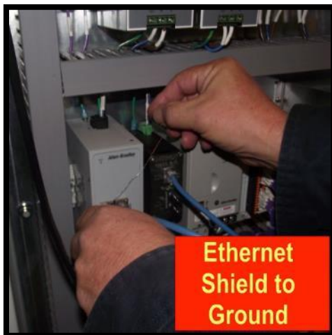
Figure 9, Ethernet Connection and Ground
