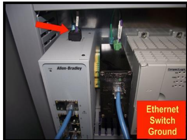
Figure 9, Ethernet Connection and Ground
