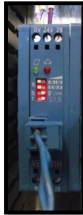
Figure 1, Safety Loop Detector
