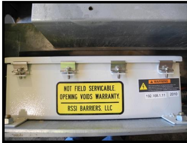
Figure 10, Servo Drive Box Inside Barrier
