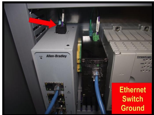
Figure 2-11, Ethernet Connection and Ground
