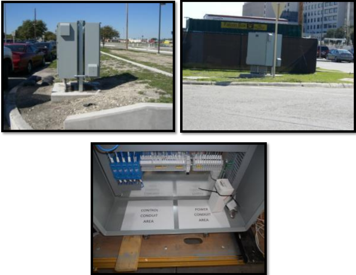
Figure 2-7, EPU Control Panel & Battery Back-up
