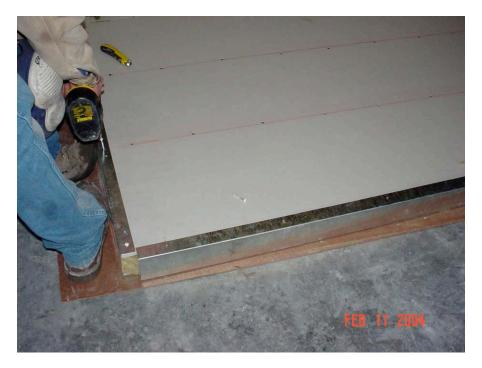
The channel was attached at each stud location with 1-1/2" laminating screws
