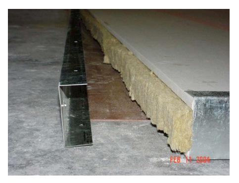
3", 20 GA channel installed around the perimeter
