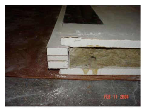
Gypsum filler installed at a panel connection
