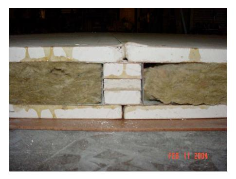
Gypsum filler installed at a panel connection
