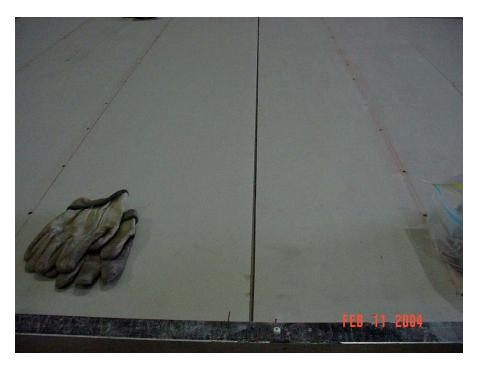
Panel joint prior to installing cover
