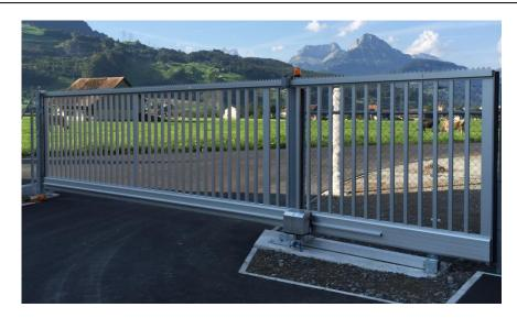
Design: Power-operated cantilever sliding gate with electro-mechanical drive, control
