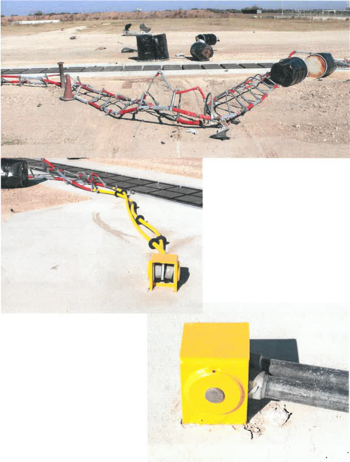
Figure 7. Installation after test 400001-USR22.
