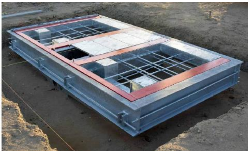
Figure 3 - 828 Wedge Barrier Install
