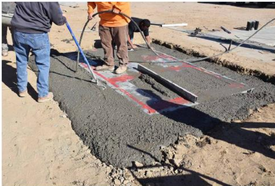
Figure 6 - Concrete Finishing
