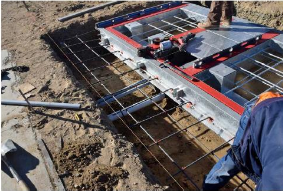
Figure 4 - Rebar install
