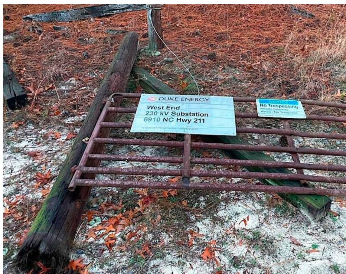
Access control measures need to be updated for current threats
