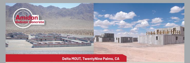
Amidon Ballistic Concrete has the distinction of building the largest ballistic live-fire facilities for the U.S. Military including the U.S. Army Delta MOUT site at TwentyNine Palms, CA. The entire project amounted to 34 buildings, 4,800 ballistic walls and 18,000 target blocks and was designed, fabricated, installed, tested and cleared for service within 270 days.
