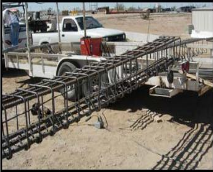
Install Pre-Assembled Side Saddle Rebar
