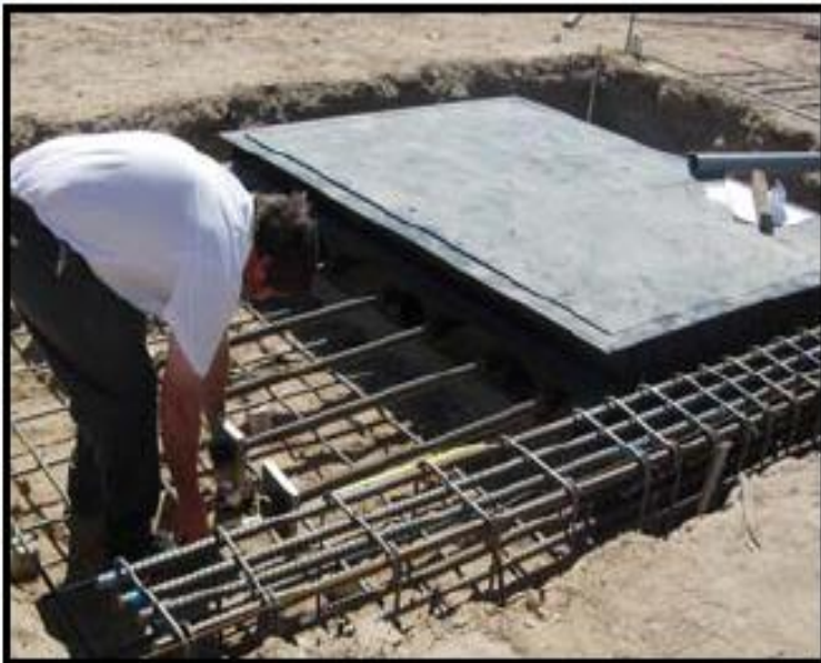
Install Pre-Assembled Side Saddle Rebar
