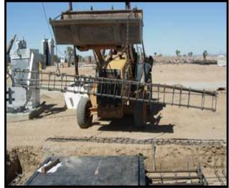
Install Pre-Assembled Side Saddle Rebar
