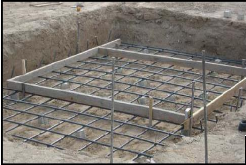
First Layer of Rebar and Concrete Forms
