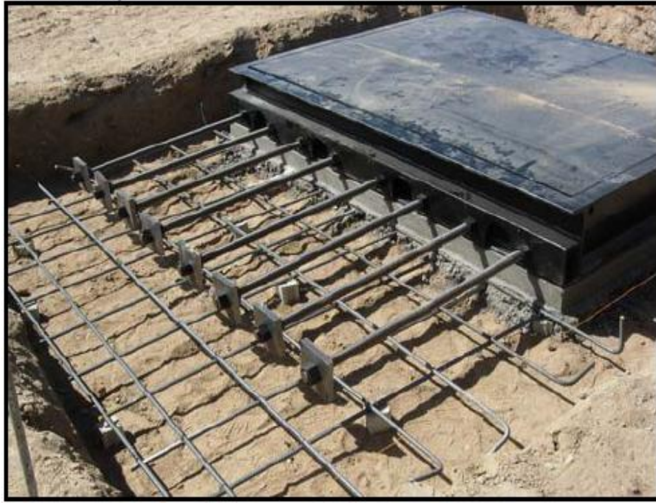
Install Anchor Bars
