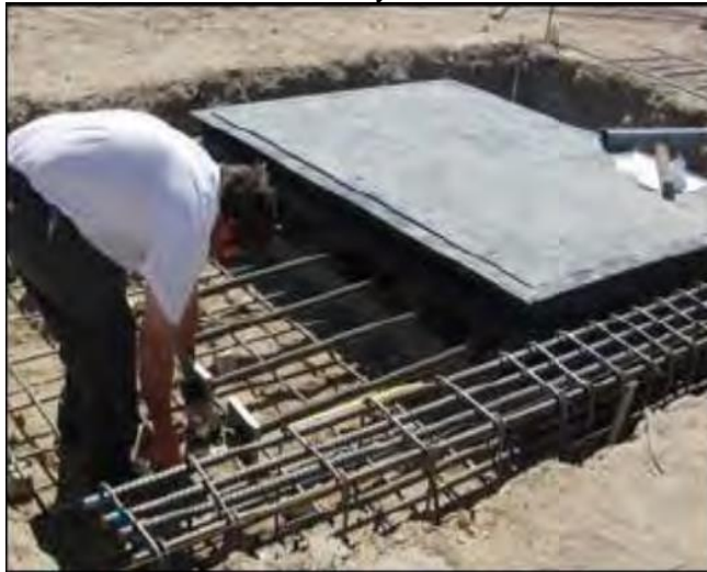
Picture 6 - Tie down Side Beam Reinforcement
