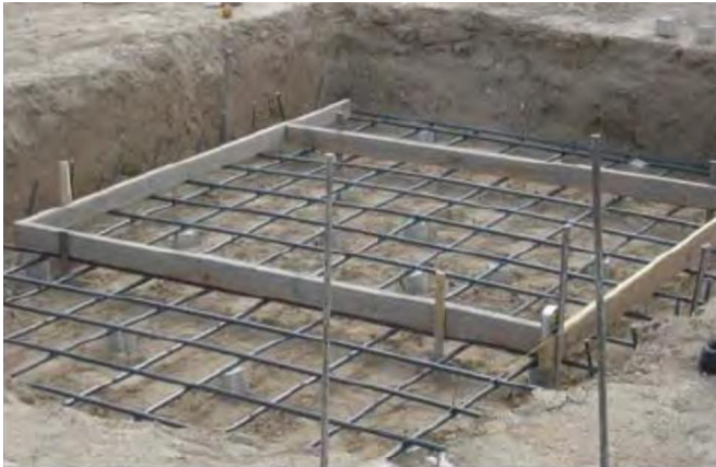
Picture 1 - First Rebar Layer / Barrier Pad Form Pad
