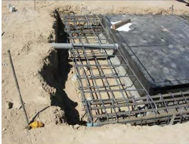
Picture 7 - Top Layer Rebar
