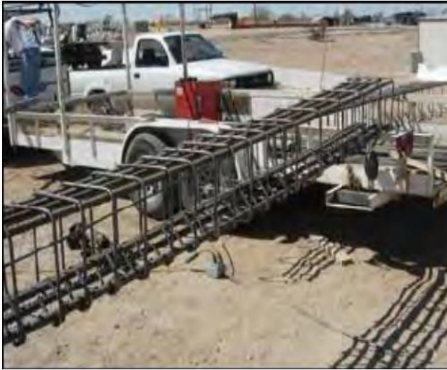
Picture 5 - Pre-Assembled Side Beam
