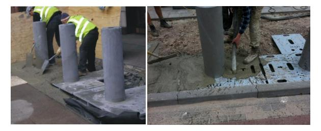
The concrete should be poured flush with top plates and biscuits and clear of excess concrete.
