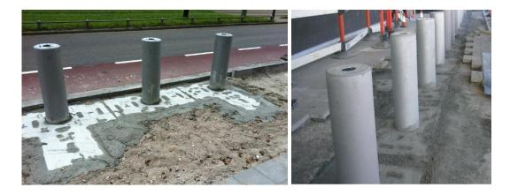
Once concrete has cured the sidewalk can be finished with appropriate materials defined by the project specification.
